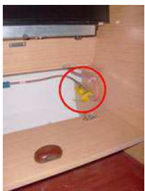
Supply valve Gas (Reference 5)
