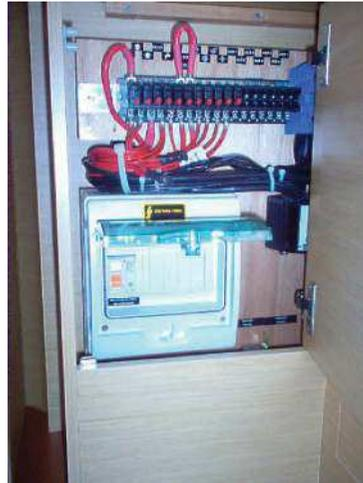
The differential switch is located in the card table
